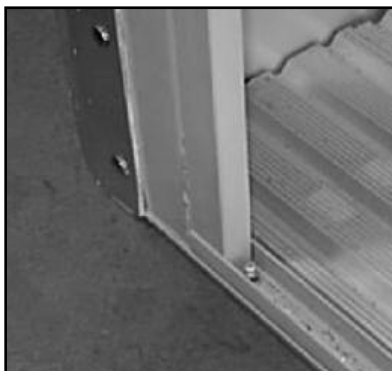
Appearance of a Huck Bolt Typical Huck Bolt Locations
